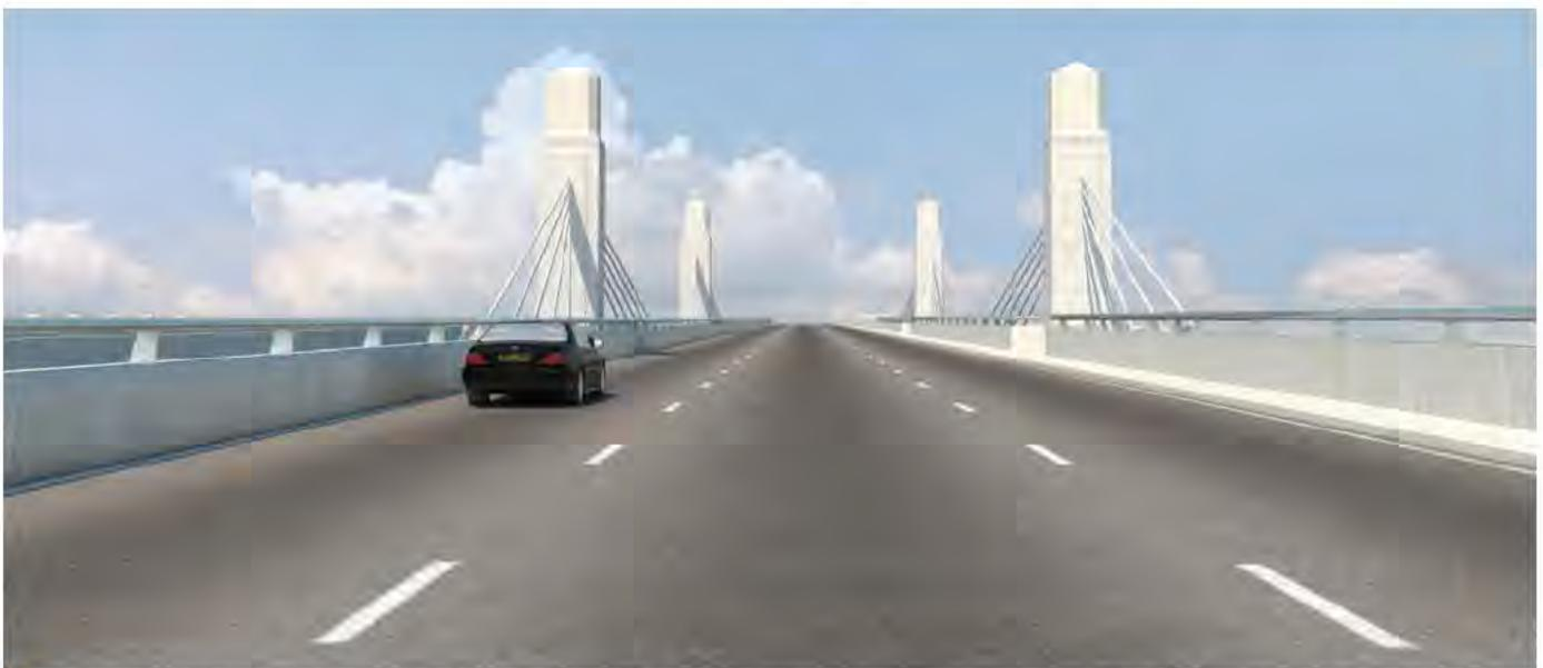
TxDOT and Waco representatives decided to create signature twin frontage road bridges on each side of the mainline bridges. Though aesthetics was certainly a driving force behind the new bridge design, the initial defining characteristic of the project was functional need.
